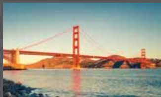
Golden Gate Bridge
